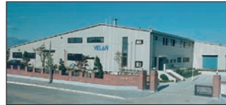
Ansan City, South Korea Velan Ltd., Plant 1
