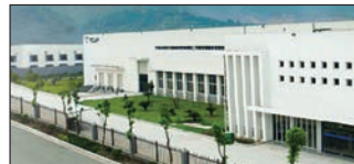
Suzhou, China Velan Valve (Suzhou) Co., Ltd.
