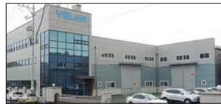
Ansan City, South Korea Velan Ltd., Plant 3
