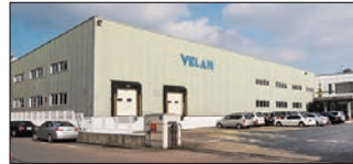
Ansan City, South Korea Velan Ltd., Plant 2
