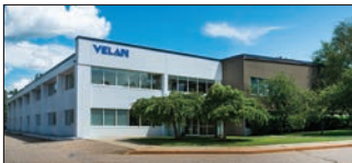
Williston, VT, U.S.A. Velan Valve Corp., Plant 3
